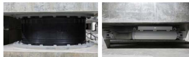
Fig 6. Location of Isolation Devices
