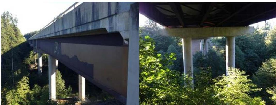
Fig. 2 – Side view of concrete deck-steel girder system (left) and piers in middle spans (right)
