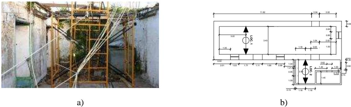
Fig. 2 - Basics of the testing layout in house 1: a) general inside view; b) plan layout and test locations.
