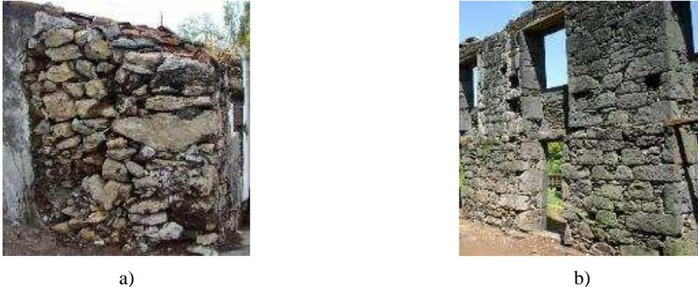
Fig. 1 - Effectively tested masonry types: a) two-leaf irregular masonry with poor fill material; b) two-leaf regular masonry with dry joints.
