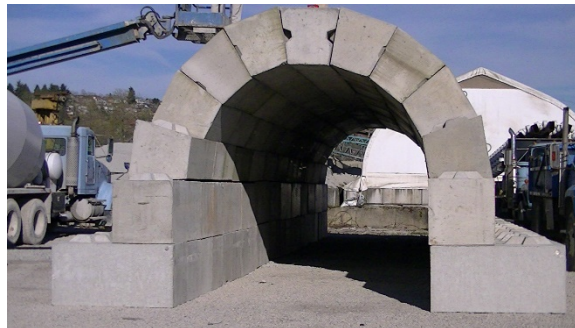
Fig. 1 – Lock-Block arch structure
