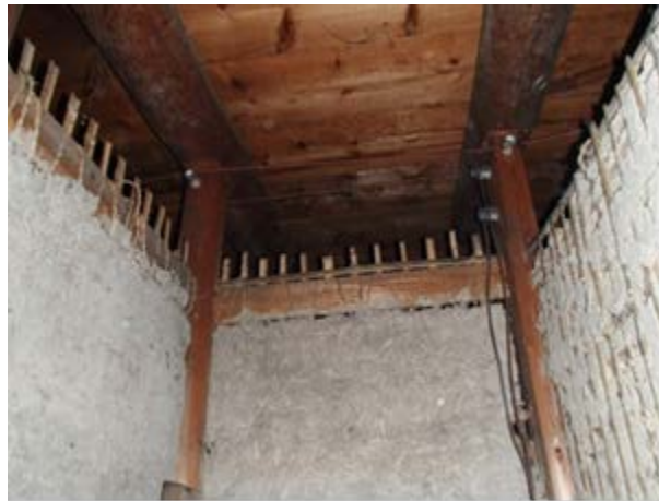
Photo 1 – Mud wall without wall clay in attic
