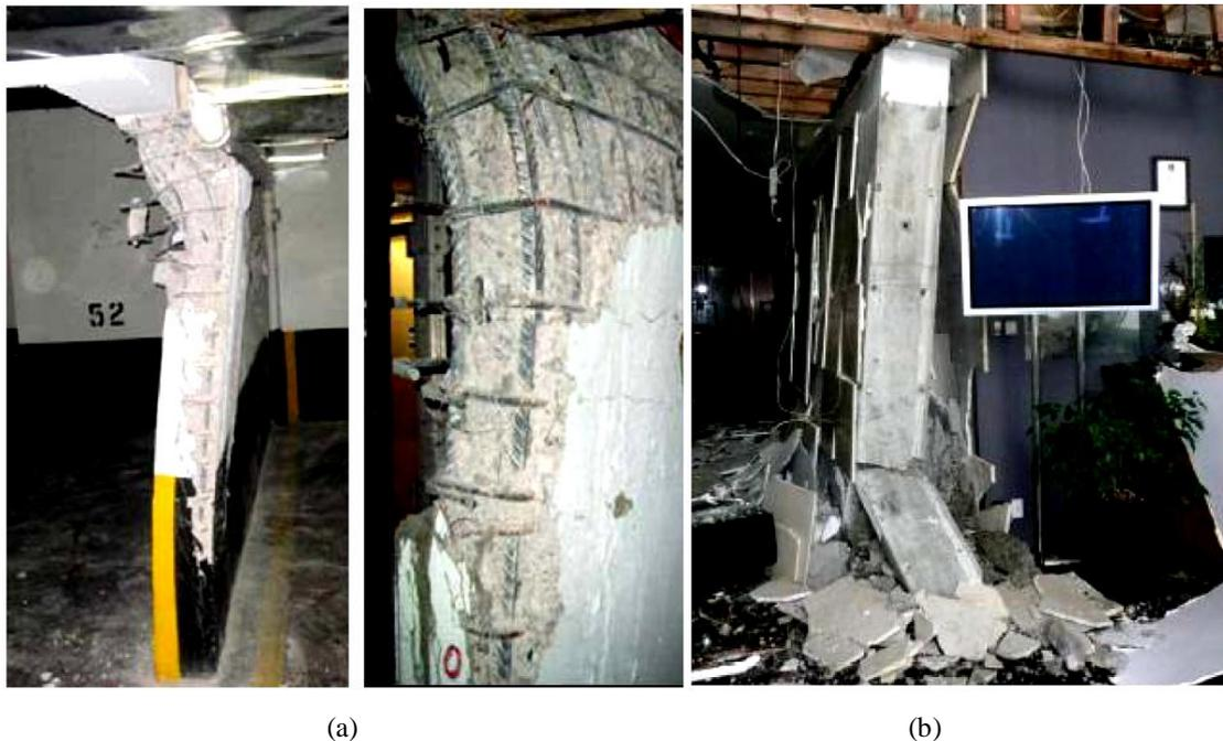
Fig. 1 – Wall failure modes observed in recent earthquakes in (a) Chile [2] and (b) New Zealand [3]
