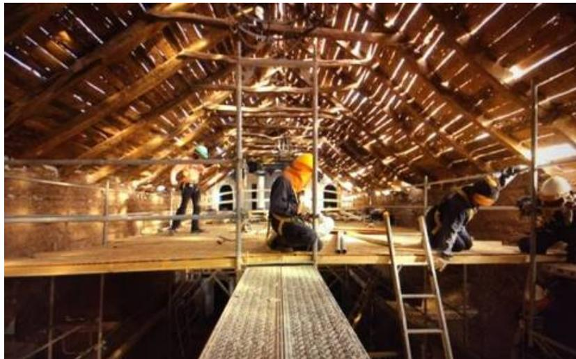
Fig. 9. Support platform to work the wooden roof.
