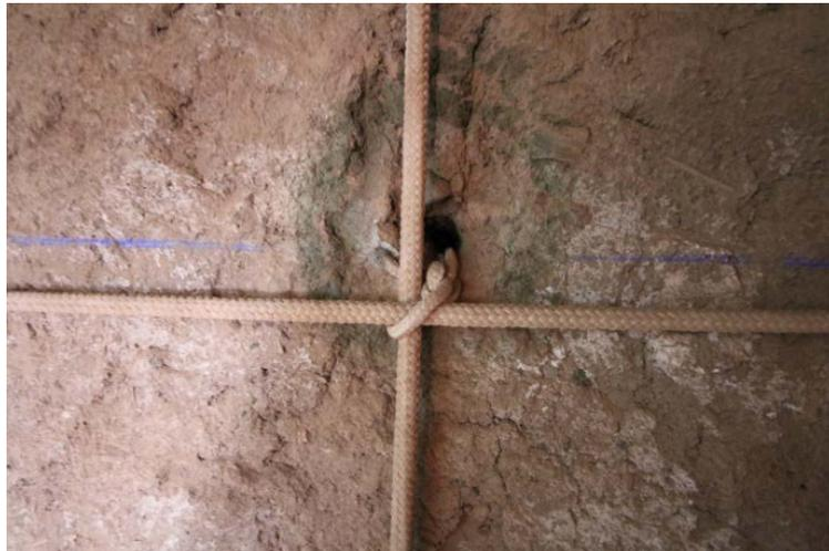
Fig. 14. Crosstie ties the ropes at the intersection
