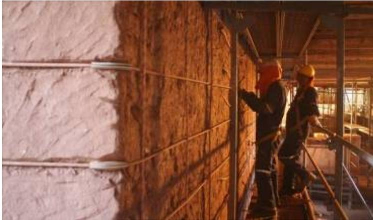
Fig. 12. Structural reinforcement by tensioning synthetic ropes.
