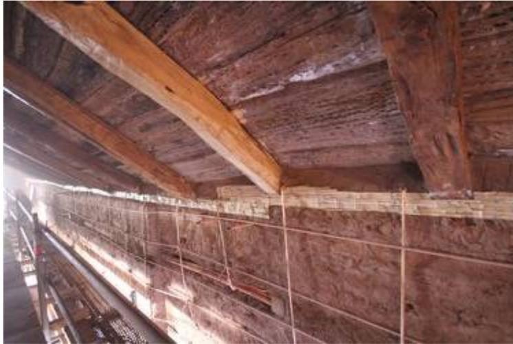
Fig. 11. Ropes are connecting roof and walls through the collar beam.
