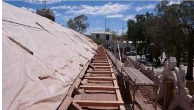
Fig. 8. Wood collar beam in the top of the walls.
