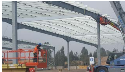
Fig. 13: Warehouse in Chile with HSS Columns and H Beams
