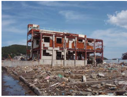
Fig. 3: Steel Frame Structure Intact
