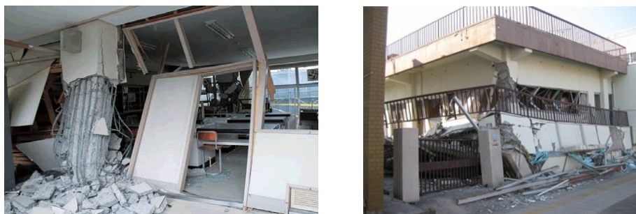
Fig. 2: Major Structural Damages on RC Structure
