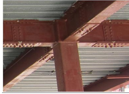
Fig. 4: No Damage with Steel Box Column to H-Beam Rigid Frame Connection
