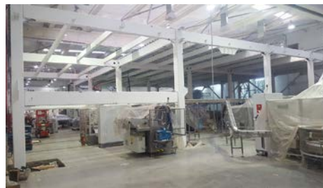
Fig. 14: Food processing plant in Chile with HSS Columns and Beams
