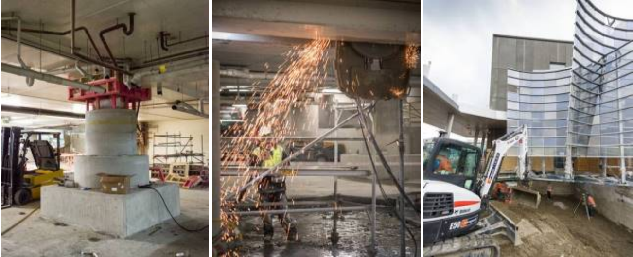
Figure 11 – a) Overhead work around columns (left), b) precision cutting works (centre) and c) temporary support works to the glazed sculptural façade (right)
