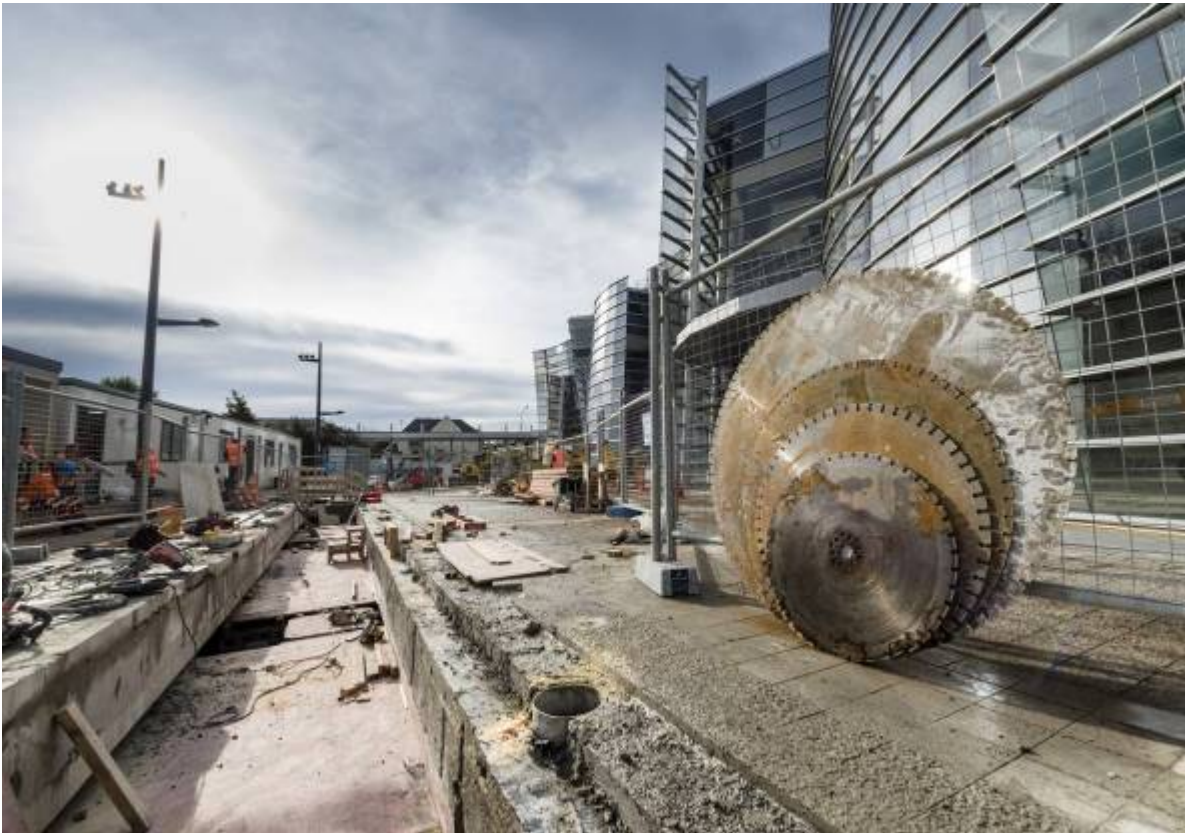
Figure 1 - Seismic trench construction adjacent to the iconic western sculptural façade
