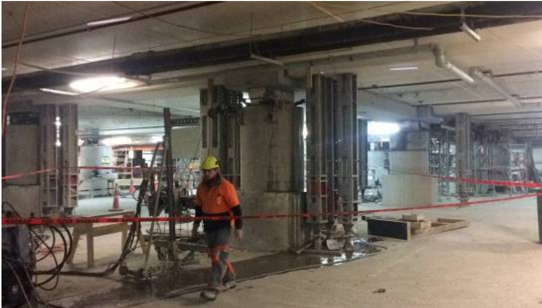
Figure 9 - A basement column being cut at the top after the mid and lower sections were jacketed and retrofitted. Propping is placed on either side of the column to allow load transfer before cutting.
