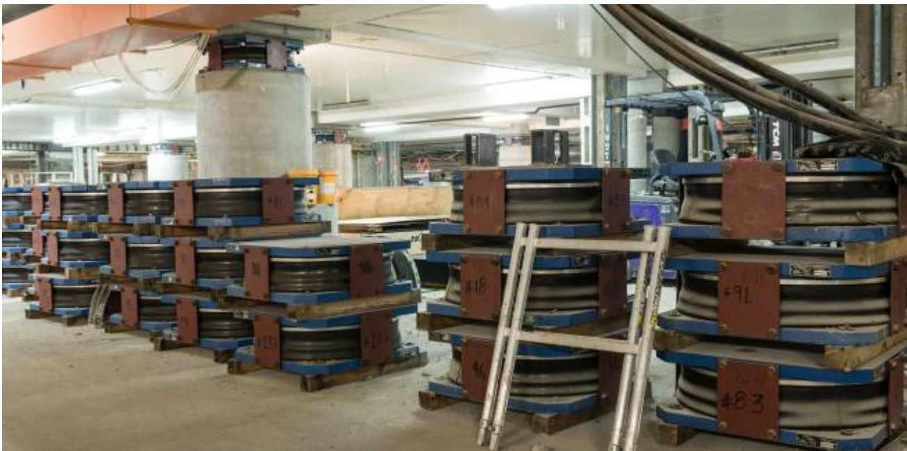
Figure 7: Triple curvature base isolation devices delivered to the Art Gallery basement for installation
