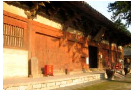
Fig.2 Great Hall of Foguang Temple on Wutai Mountain, rebuilt in 857 A.D.
