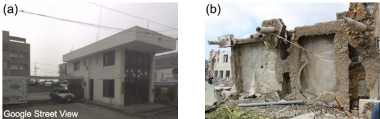
Fig. 8. Photos of Building E taken before and after the tsunami
