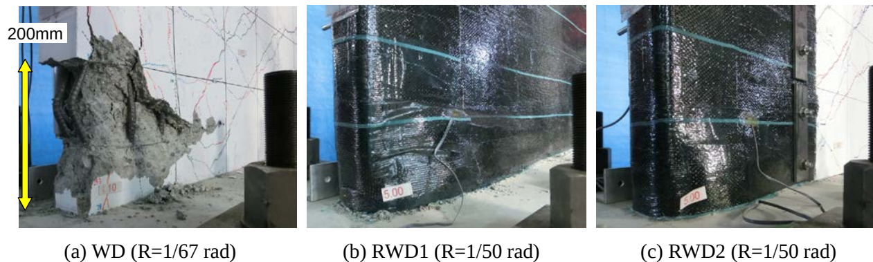
Fig. 6 – Wall base condition at failure for each specimen
