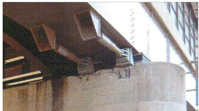
Fig.16 Nakanose Viaduct and observed damage of dampers
