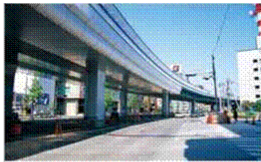
Fig.7 Benten Viaduct of Hanshin Expressway
