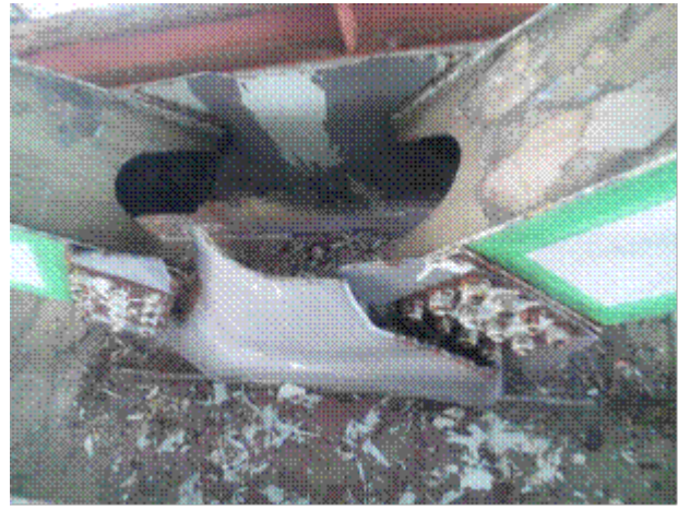
Fig.15 Damage at gusset plates of Arakawa Bay Side Bridge.
