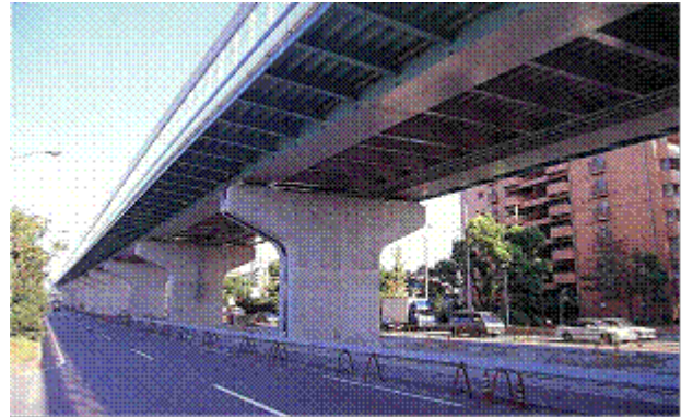
(b) reconstructed base-isolated bridge
