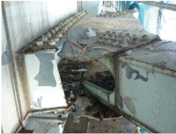
Fig.15 Damage at gusset plates of Arakawa Bay Side Bridge.
