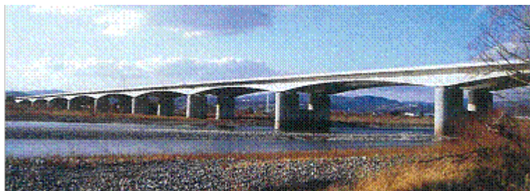
Fig. 8 Tenryu River Bridge
