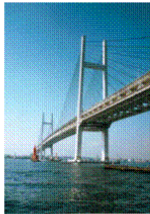
Fig. 10 Yokohama Bay Bridge
