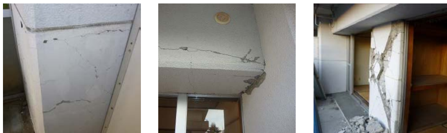
Fig. 4 – Typical damage to the columns, beams, and nonstructural walls
