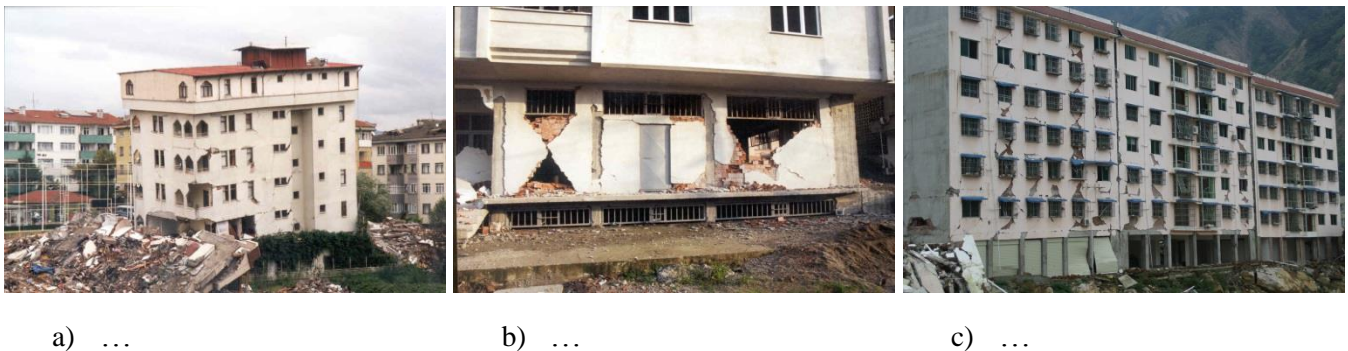
Fig. 1 – Different levels of damage of different height reinforced concrete frame buildings with URM infill walls [11]
