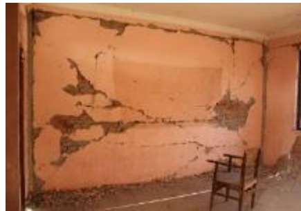
b) Infill shear and minor frame damages, Nepal 2015
