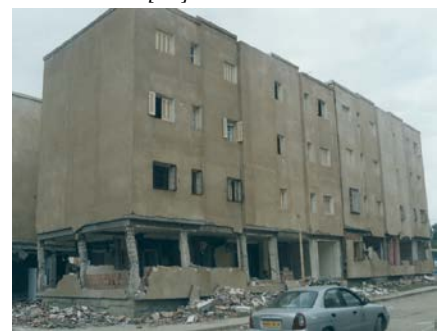
f) Damage to an apartment building with a soft first storey in Bordj-Kiffan city, Algeria 2003 [14]
