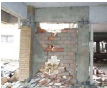
a) Infill shear and major frame damages, Chania 2008 [10]
