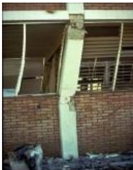
d) Captive column failure, Managua 1972 [12]
