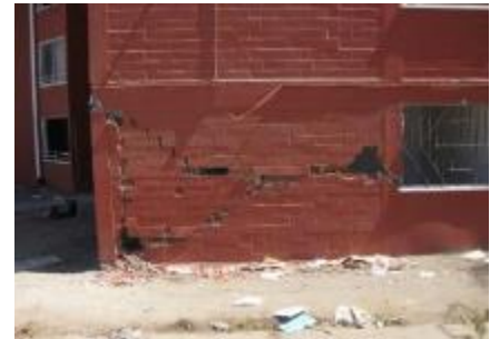
c) In-plane shear failure in infill and shear failure at the ends of RC column, San Antonio 2010 [11]
