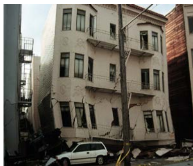
e) A collapsed soft storey apartment building in the Marina District, San Francisco 1989 (Loma Prieta Earthquake) [13]
