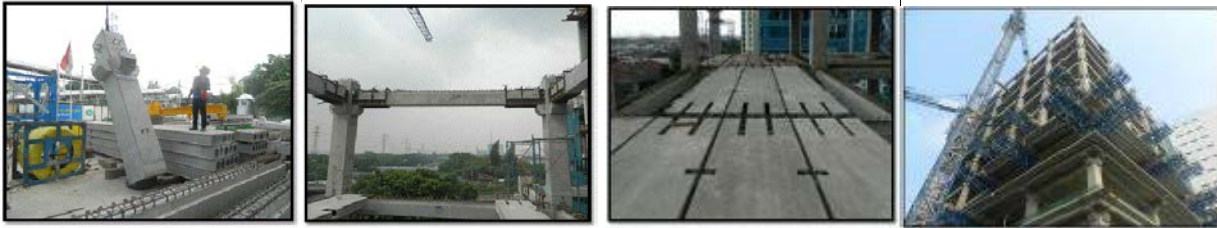
Fig.19 – Application in twelve storey office building in Jakarta
