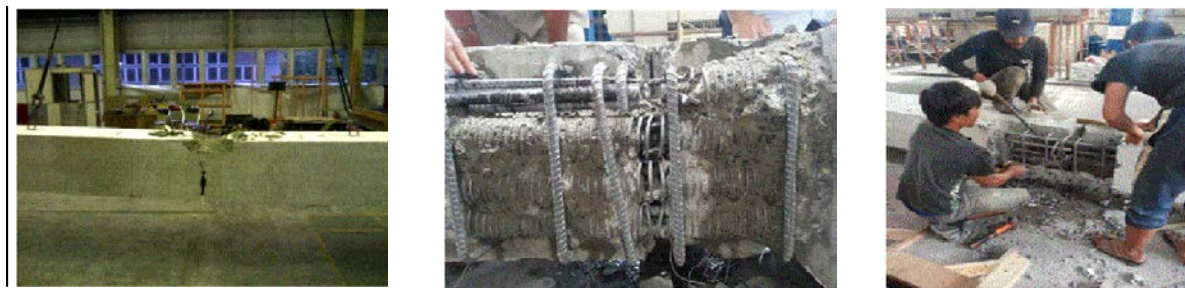
Fig. 14 – Repair of precast segmental hybrid beam and connected with new dissipater ( A_s/A_s' = 1.14 )
