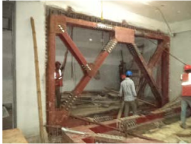
a) A steel braced frame at inside (a storage area)
