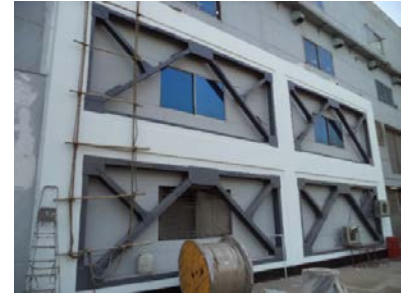
c) Steel braced frames at perimeter
