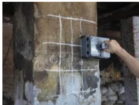
Photo A.2- Location and size of rebar
