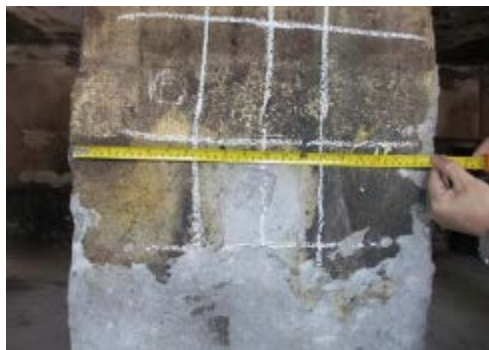
Photo A.1- Measuring by scale (column)
