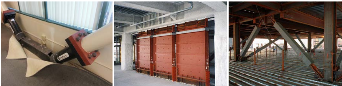
Fig. 1 – Supplemental energy dissipation devices: FVDs, VWDs, BRBs from left to right
