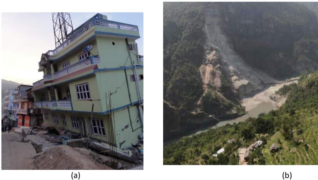
Fig. 1 – (a) Complete collapse of ground floor of a multistory reinforced concrete frame with infill masonry wall construction on slopes due to soft story effect coupled with ground failure (photo by Kishor Jaiswal at the U.S. Geological Survey); and (b) Rock slide along the Kali Gandaki River (reproduced from [1]).
