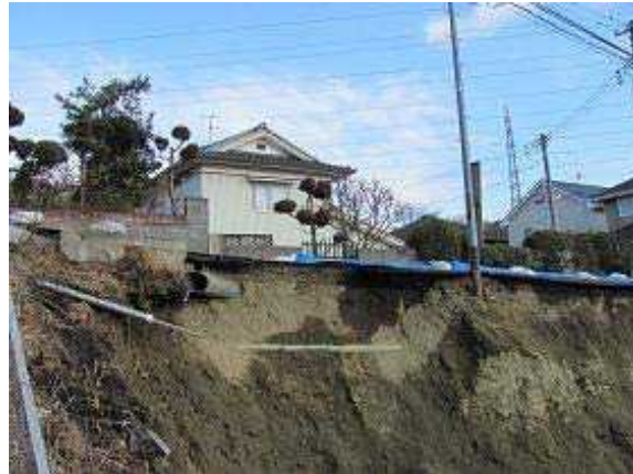
Fig. 1 – Exposed welded steel pipe owing to slope failure [1]
