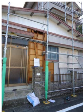
Fig 3— Seismic retrofit, Example 1
