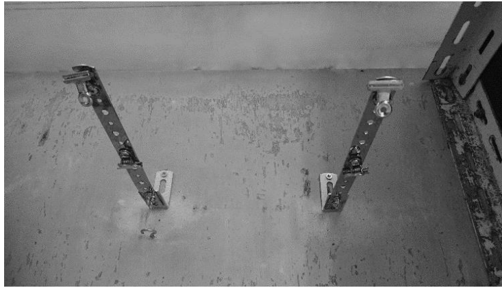
Fig. 6 – Steel mounting plate for the water pressure gauge
