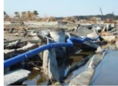
Photo 3 - Damage to pipe by tsunami-induced scouring
