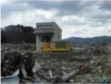
Photo 1 - Inundated intake facilities (Sukedukuri No.2)
