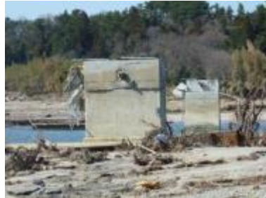
Photo 2 - Washed-away water pipe bridge
