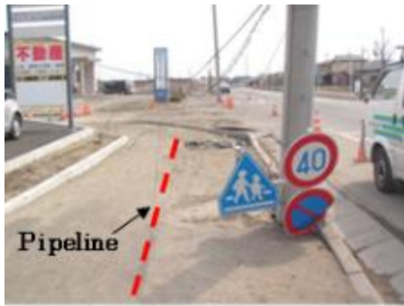
Photo 6 - Subsidence of utility pole induced by liquefaction in Sendai City
