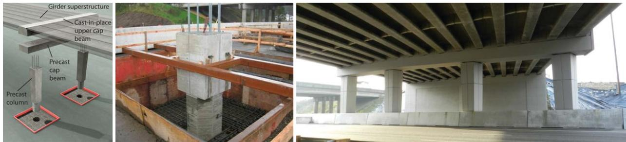
(a) GDC and MSC in a bent      (b) Column to footing MSC      (c) Completed bridge
