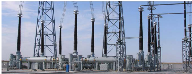
Fig. 1 – GIS used in substation
