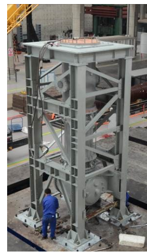
(b) The construction of Frame-R
