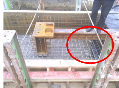
Fig.10 – Pit with framework
