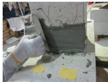
(a) Rebuilding of damaged cross section with PCM
