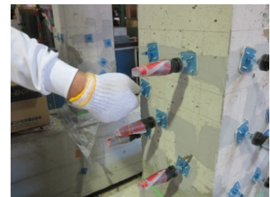
(b) Injection of epoxy resin
