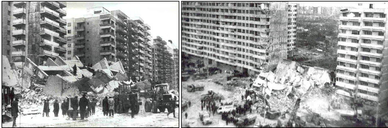
Fig. 5 – Images of the section “F” that collapsed (AGERPRES)
