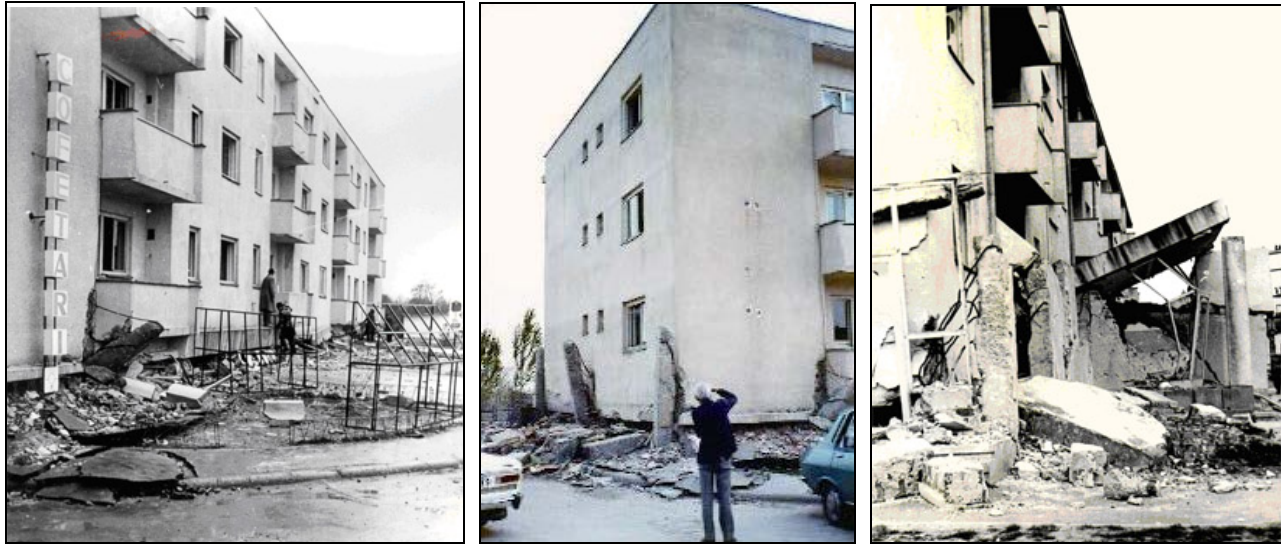
Fig. 9 – The “Valea Călugărească” building with its “vanished” ground floor (ICCPDC-INCERC and JICA)
