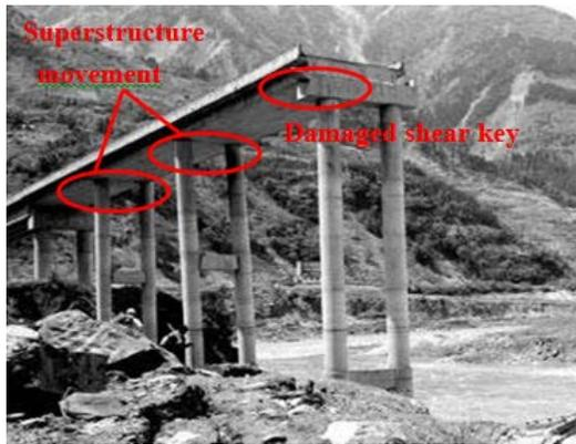
(a) bearings slipping and damaged shear key
