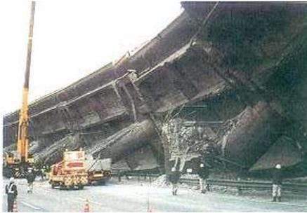
Fig. 3–Pier damage in Kobe viaduct bridge
