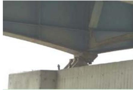
Fig. 4–Failure mode of bearings
