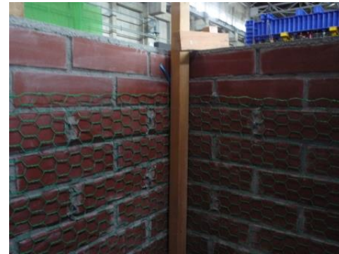
(2)Wall before with Floor working
