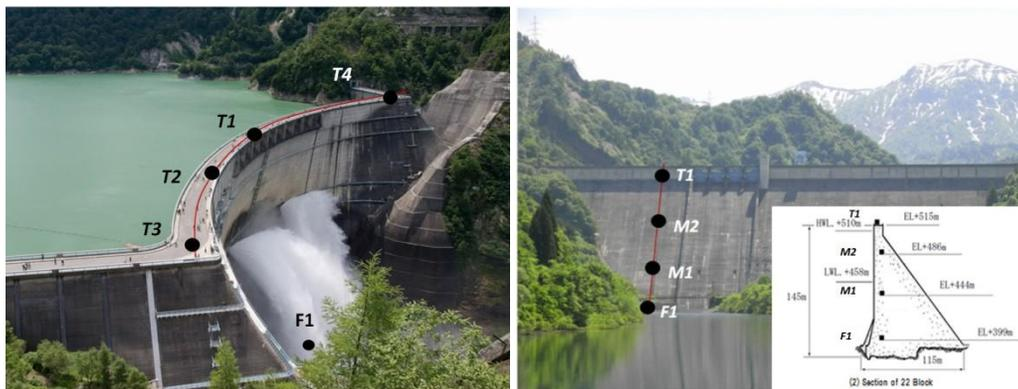
Fig. 1- Kurobe arch dam (left) and Tagokura gravity dam (right) sensor's location
