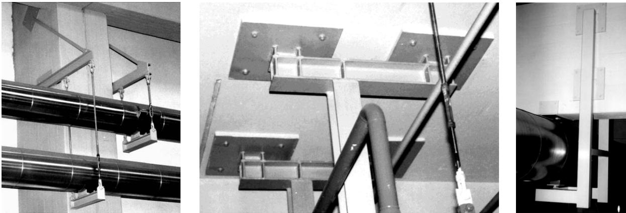
Fig. 1 – Post-installed anchorages of piping systems [1]
