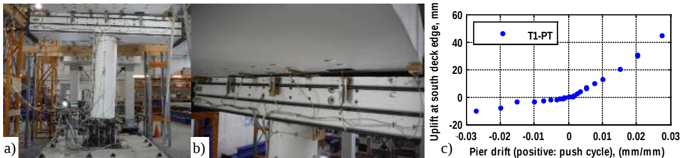
Fig. 11: a) Pier deformed shape at 2% drift (push phase); b) Close up of gap opening between deck and cap beam at 2% drift (push phase); c) Measured deck-cap beam uplift at the southern edge of the deck.
