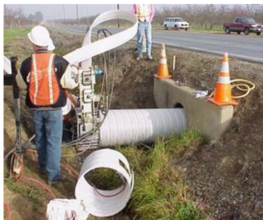
Fig. 1 CIPP lining technology (a) pipeline rehabilitation with CIPP liner (b) cross-sectional view of push-on joint of a ductile iron pipeline reinforced with CIPP liner-
