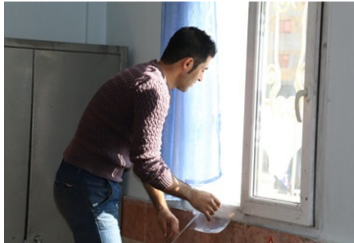
Fig. 5 – Using glass tapes on all windows to protect people from potential injuries
