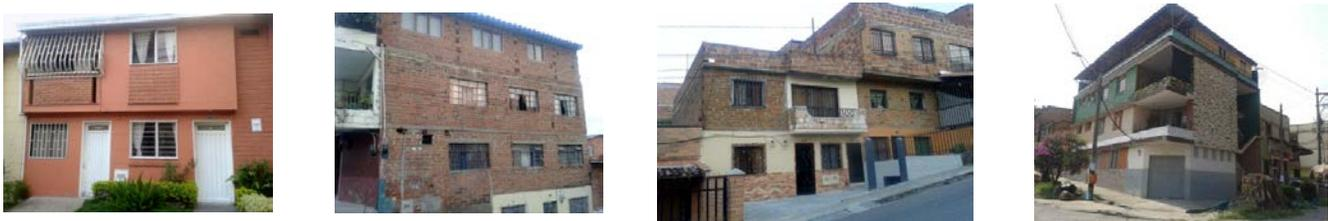
Fig. 4 – Examples of unreinforced masonry structures of Medellín
