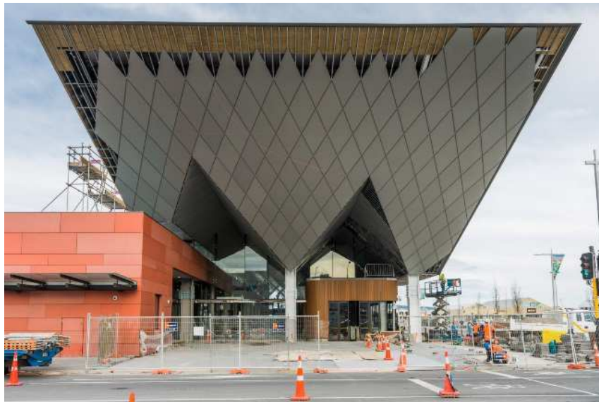
Fig. 3- CBI Main Entrance Corner Cantilever under construction (Site photograph courtesy of Aurecon New Zealand).
