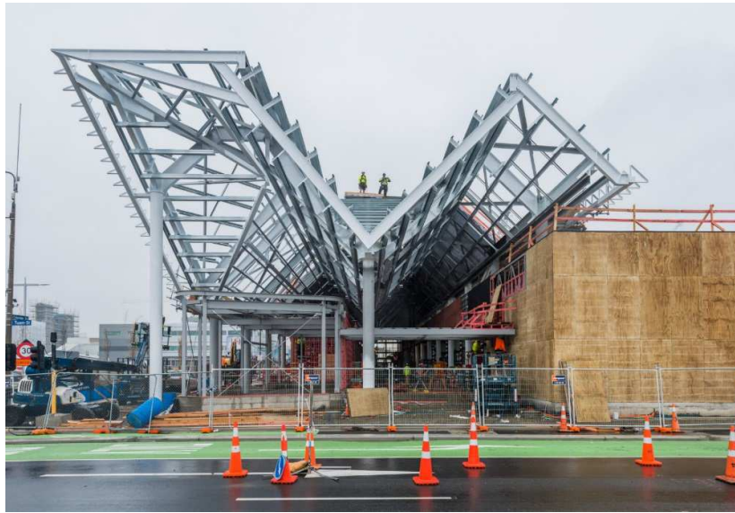
Fig. 6- Image of the Christchurch Bus Interchange South Elevation under construction (Site photograph courtesy of Aurecon New Zealand).
