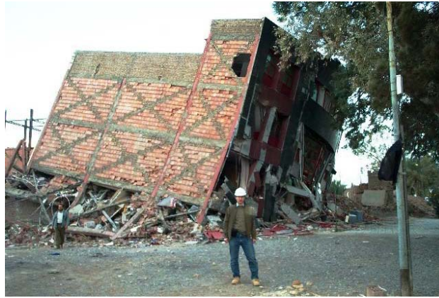
Fig. 2 – Damaged building due to mass and stiffness eccentricity Bam Earthquake, 2003 [6]
