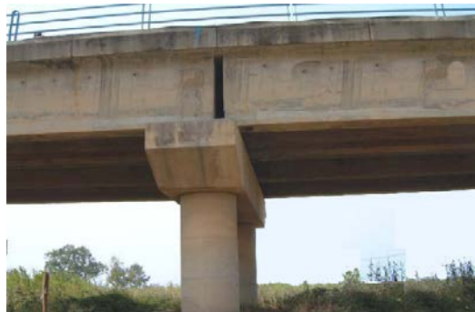
Fig. 8 – Girder displacement of Sebaou Bridge
