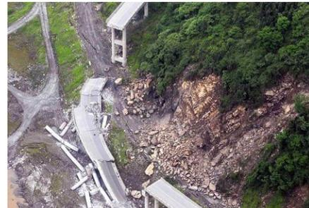
Fig. 5 – Collapsed spans in unit 5 after demolition
