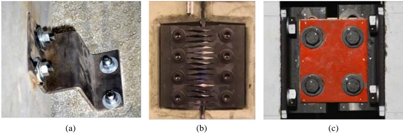
Fig. 4 – View of the dissipative panel connections: (a) FPD; (b) MSD; (c) FBD.
