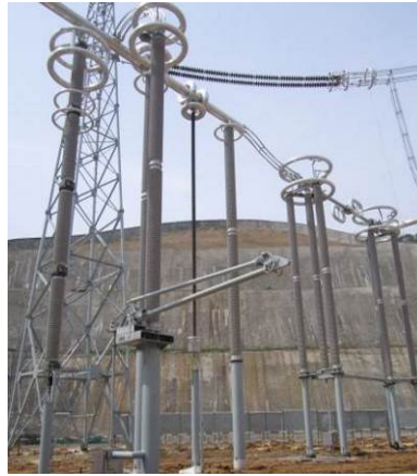
Fig. 3 Electrical equipment assembled with composite insulator in substations
