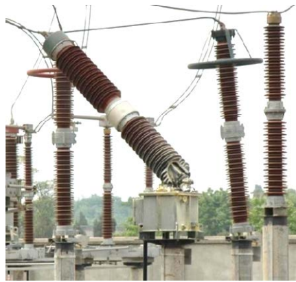
Fig. 1 Failure of porcelain insulator in 2008 Wencuan earthquake
