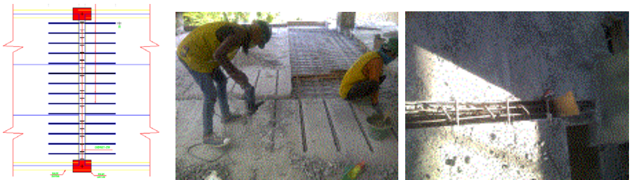
Figure 11 – Extra reinforcement for floor slab
