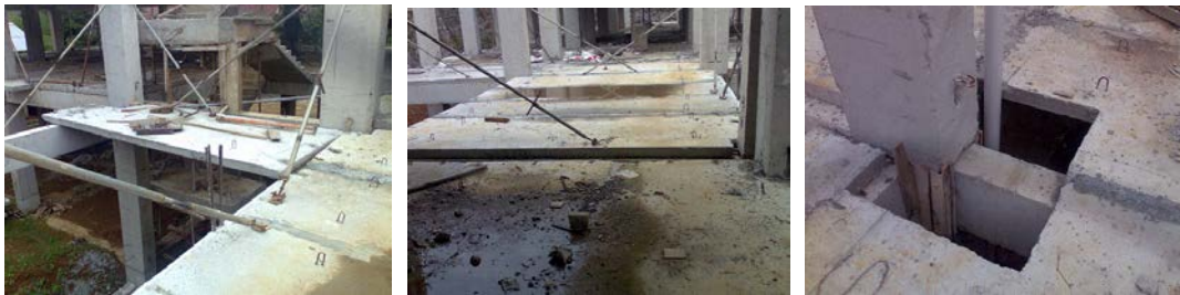
Figure 6 – Beam-slab joint condition at field
