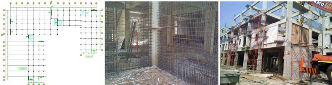
Figure. 9 – Location and reinforcement of shear wall
