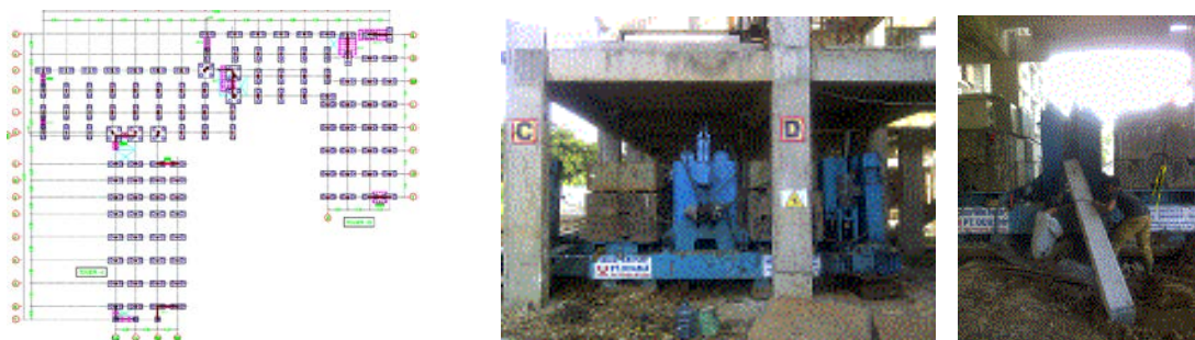
Figure 10 – Additional foundation at shear wall base
