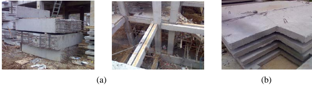
Figure 3 – Condition of beam and column components
