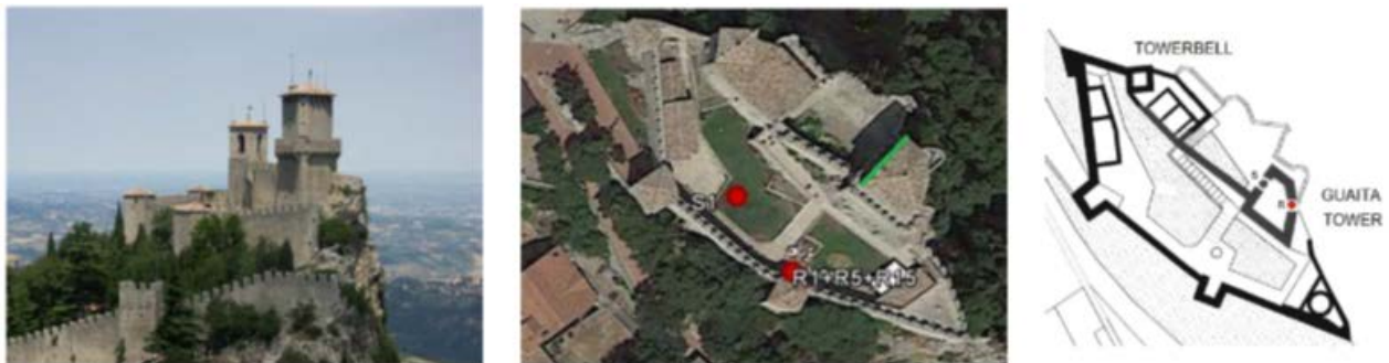
Fig. 2 – Guaita Tower and location of the measurements performed outside and inside the building. The green line indicates the direction of the walls assumed as reference (NS component). With the grey circle are indicated the measurements performed with an instrument, with the red one the measurements performed with the other one.
