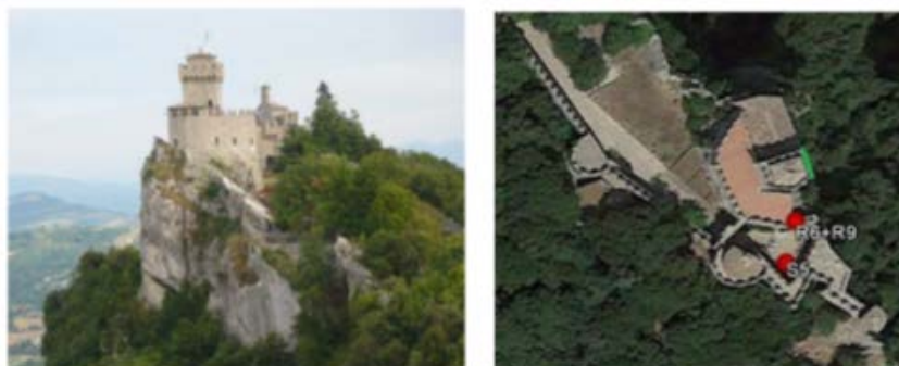
Fig. 3 – Cesta Tower and location of the measurements performed outside the building. The green line indicates the direction of the walls assumed as reference (NS component).
