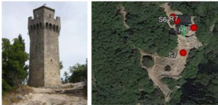
Fig. 5 – Montale Tower and location of the measurements performed outside the building. The green line indicates the direction of the walls assumed as reference (established NS component).
